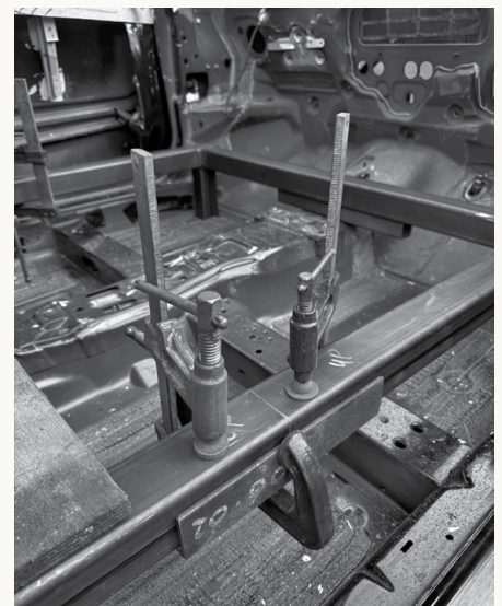
Welding the subframe. Skilled craftsman, Mick Bennett, at Blackwater, welded a new 40mm box section steel chassis to the existing folded steel monocoque structure. ©David Cotterrell
